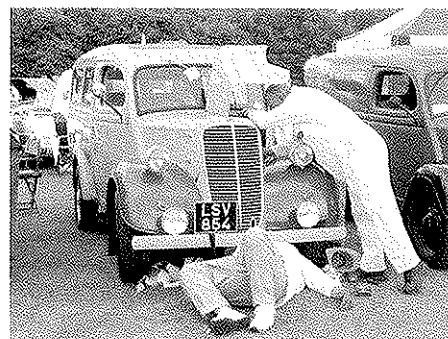
Dave Rothwell (white overalls) and Ron Taylor supervise Dave Broad changing the fuel pump on his Utilicon.
